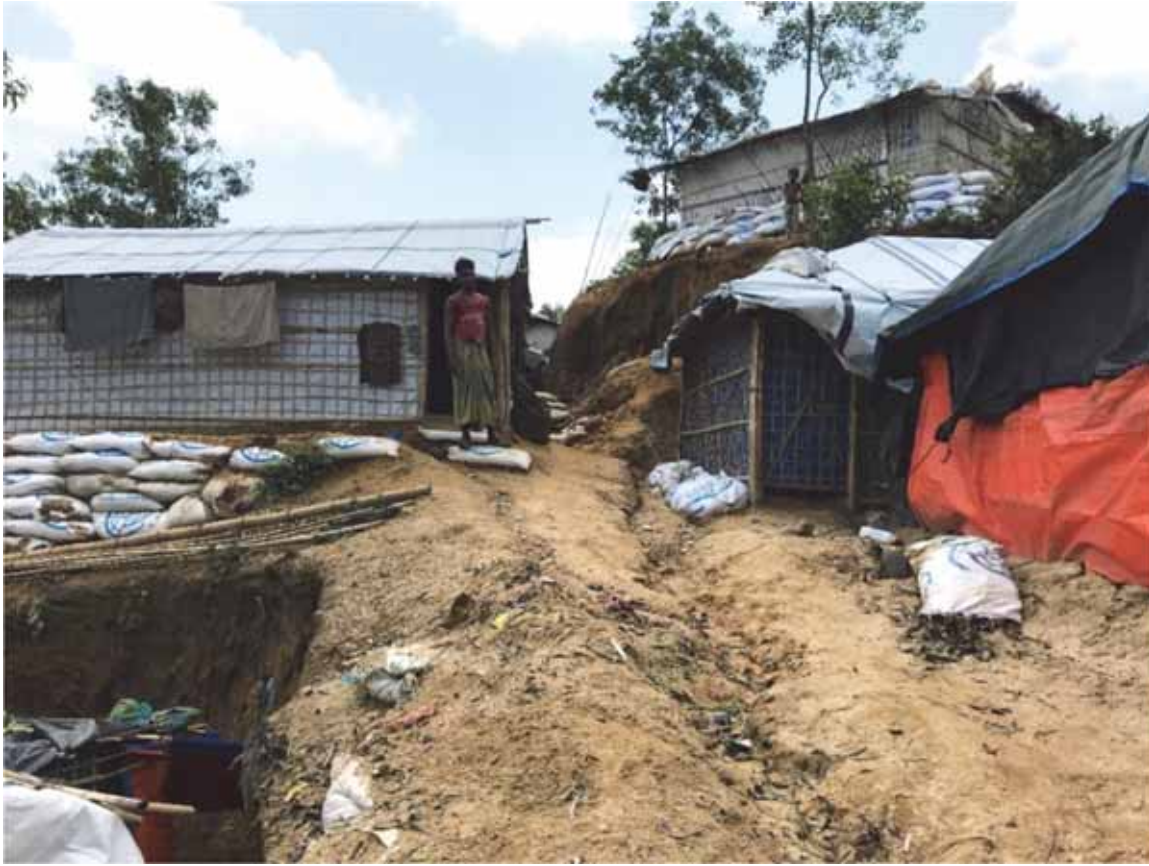
Especially when it rains, eroded gullies and lack of steps and handrails make for treacherous walking in the Kutupalong-Balukhali Expansion Camp in Cox's Bazar, Bangladesh, May 2018. Photograph by Bill Frelick. © 2018 Human Rights Watch
