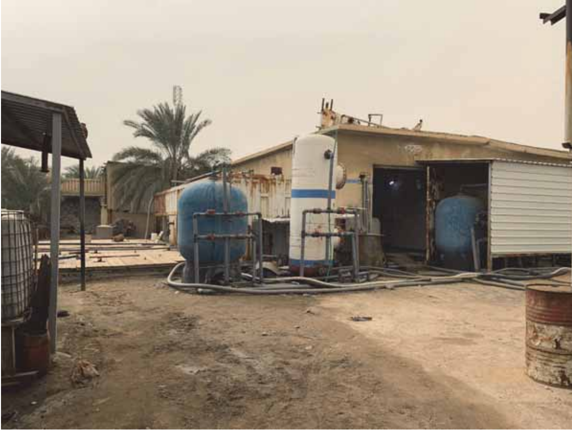
A private reverse osmosis (RO) desalination and filtering plant that sells drinking water to Basra residents. © 2019 Belkis Wille/Human Rights Watch.
