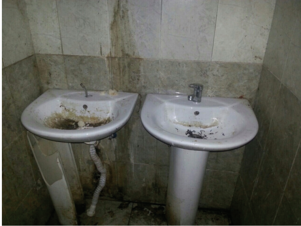
Toilets at Gazi Baba detention facility. Photo taken by a former detainee. February 2015.
